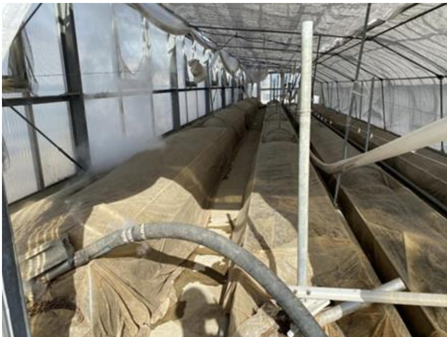
Figure 2.8 Soil in a greenhouse being steam-sterilised
